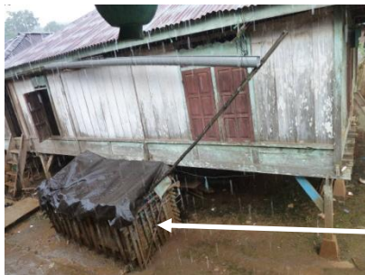
A water tent situated by the house, functioning to collect rainwater.
